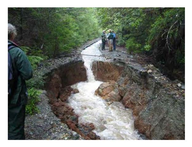
Stream Diversion due to plugged culvert on abandoned road. *Source: U.S.D.A Forest Service.*
