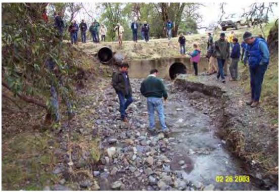
Figure 1. Example of a critical culvert installed at a stream crossing with diversion potential (Pacific Watershed Associates Inc. 2003).
