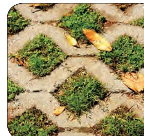
**B** Turf block works well for allowing water to SINK into the soil in medium-traffic areas or driveways with separate parking areas (pages 39).
