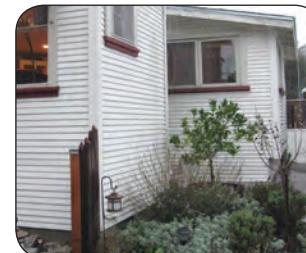
**B** Vegetated or rock drip-line protection SLOWS runoff thus reducing erosion and promoting infiltration. It is also designed so that the ground slopes away from the home's foundation (see page 27)
