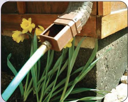
**SPLASH GUARDS** are simple devices that reduce the initial force of the water at the outlets and allow it to SPREAD out into an area of vegetation or an appropriate infiltration area and SINK back in to the soil.
