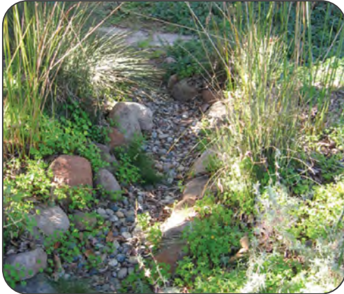
Dry creek infiltrates and conveys runoff.
