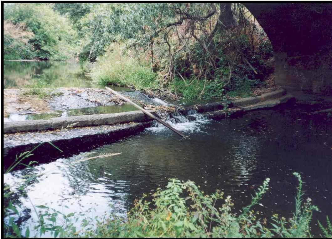
**Station Suisun Creek 4 (SC4) — Note cement drop structure under bridge**
