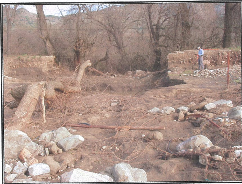
Levee break and destroyed vineyard near Yountville. (Gin)
