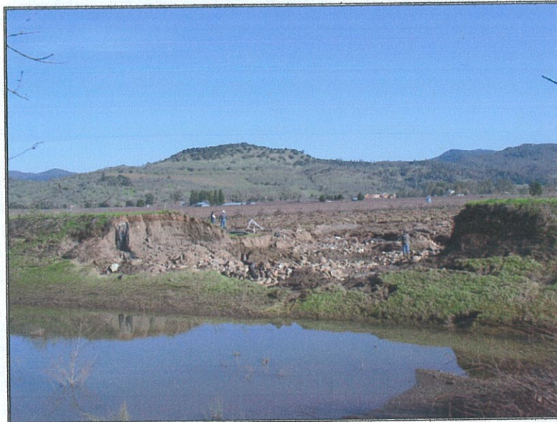
Levee break along the Napa River, near Rutherford
