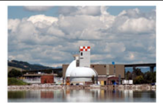
Soscol Water Recycling Facility collects and recycles methane gas for power production.
