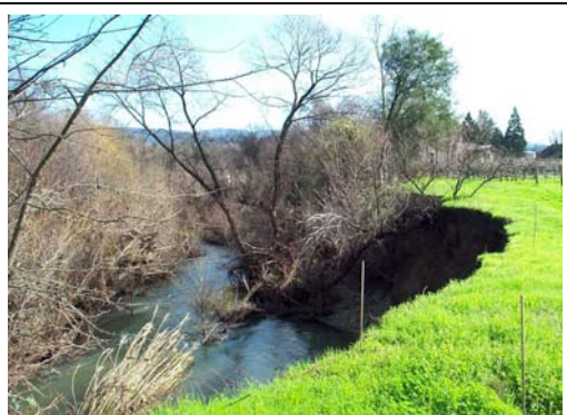
An Eroded Streambank
