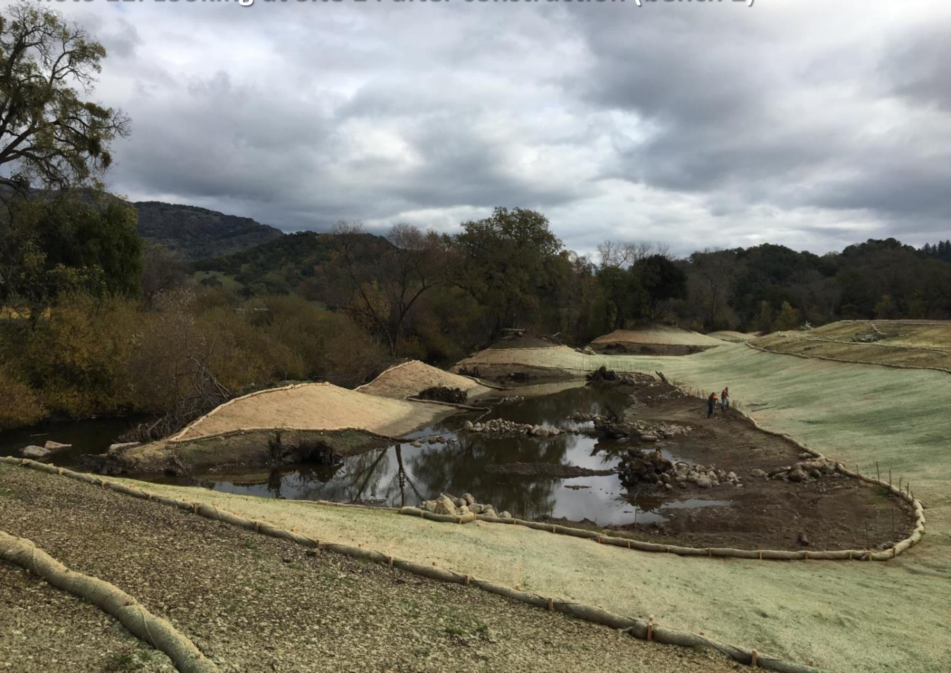
Photo 11: Looking at Site 14 after construction (bench 2)
