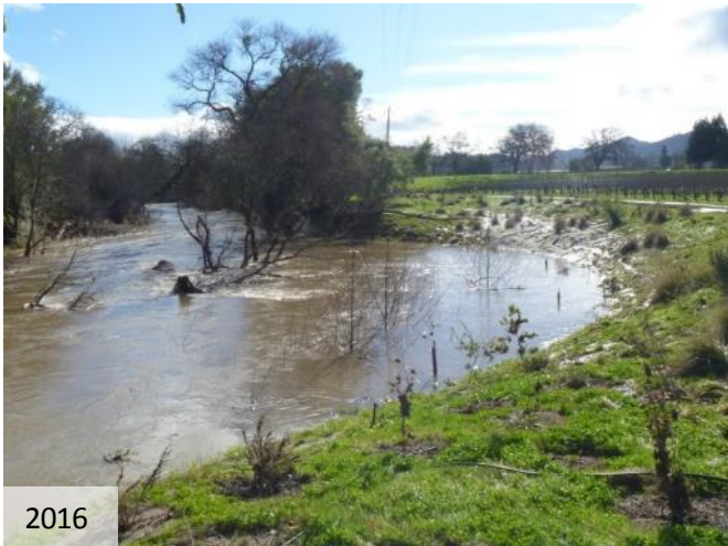
Reach 9 Bank Stabilization Site
