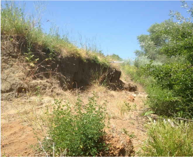
Picture 1: Bank Erosion Site Reach 3
