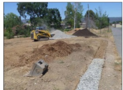
Swale built to sink stormwater from parking lot and nearby buildings
