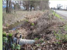
Culvert outfall, plantings at Yountville Collector
