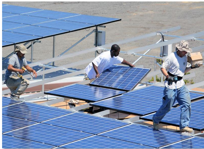
San Rafael Airport 972kW Feed in Tariff Project (Condition One)
