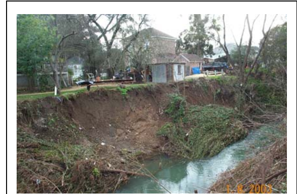
Erosion is the general process by which materials are loosened, dissolved, or worn away. There are many natural and human-related causes of erosion. The process of in-stream channel erosion, as shown in this image, includes bank slumping and shearing, channel bed incision, and channel widening.
