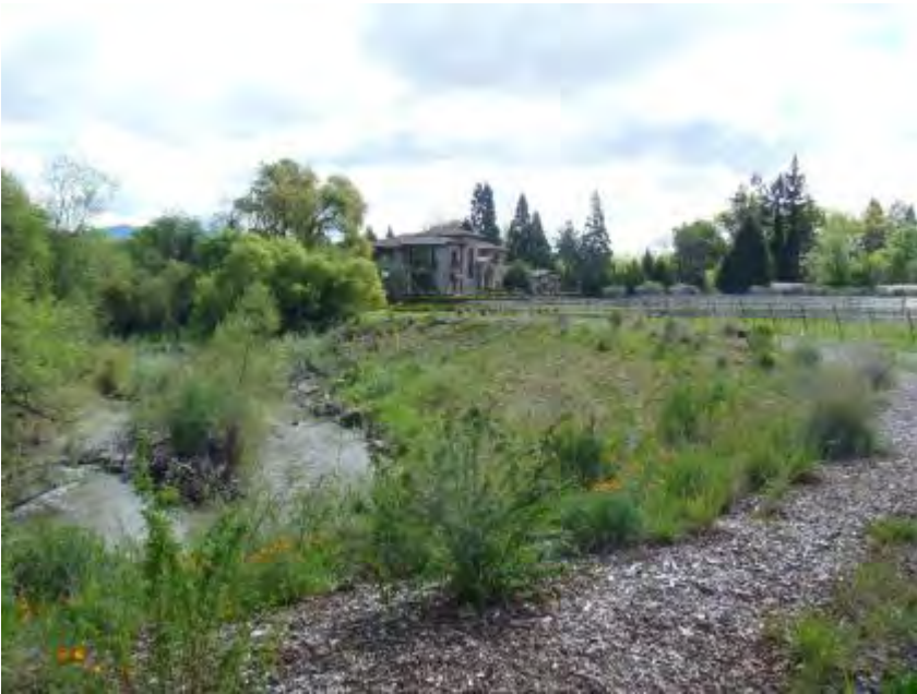
Sequoia Grove Bank Stabilization, Reach 8 North (April 2014)
