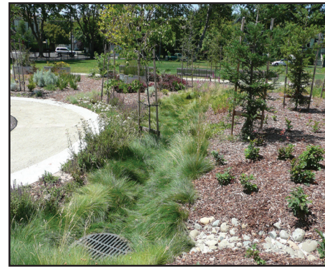
Rain garden with overflow drain at New Technology High School.
