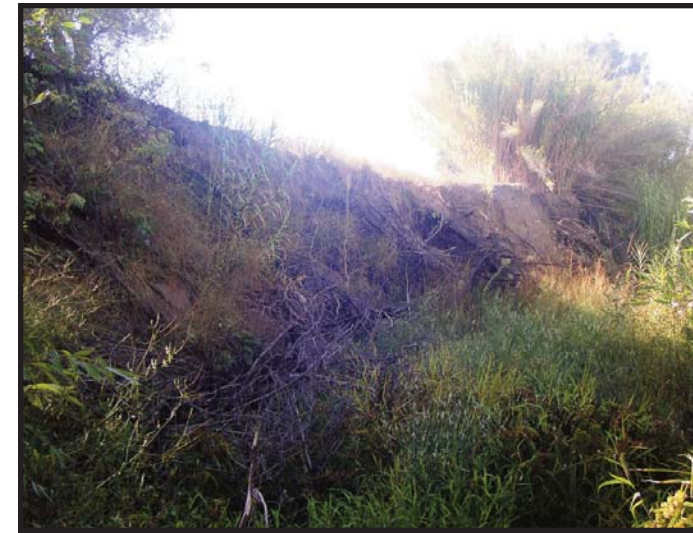
Reach 5 has several areas of vertical, eroding banks with riprap.
