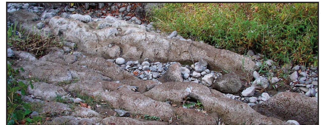
RESISTANT CLAY LAYER IN THE CHANNEL OF REACH 1
