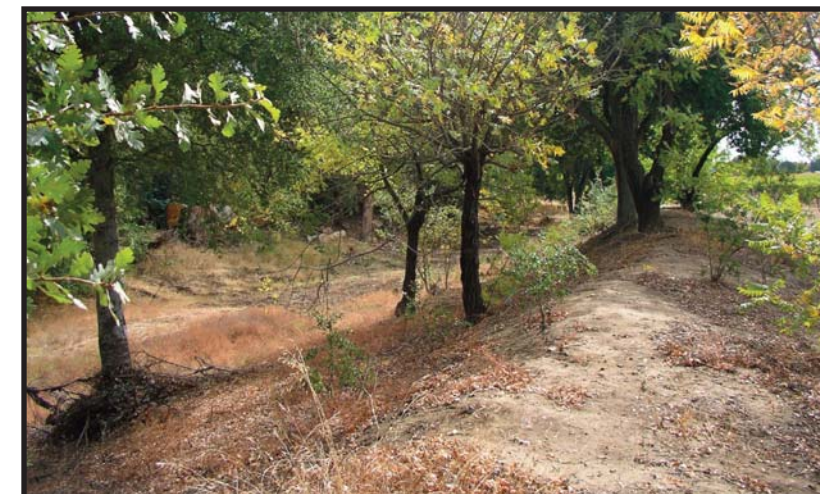
THE FLOOD CONTROL BERM IS ON THE RIGHT AND THE OVERFLOW AREA ON THE LEFT IN THIS PHOTO WITH THE RIVER CHANNEL TO THE FAR LEFT.
