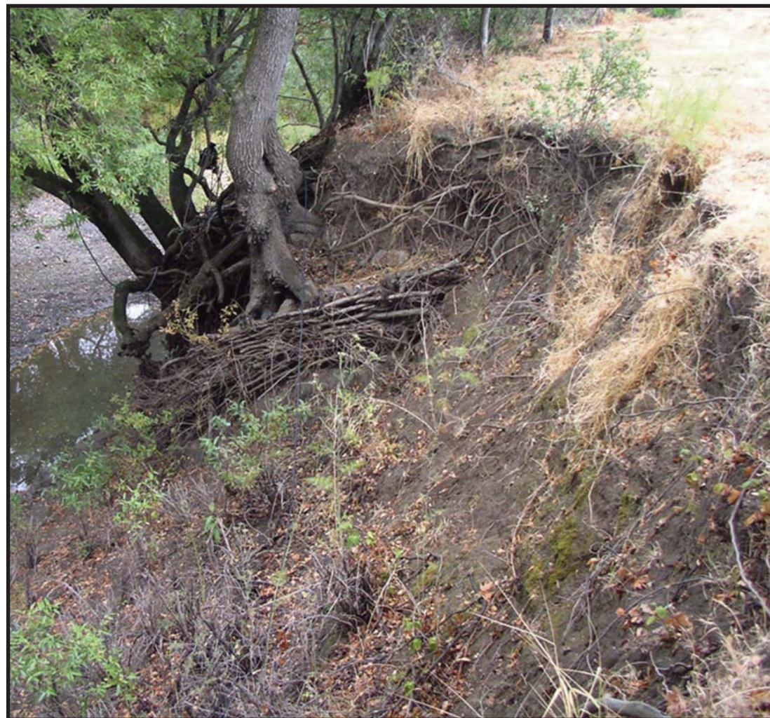
NATURAL BANK RETREAT IN RESTORATION AREA 23
