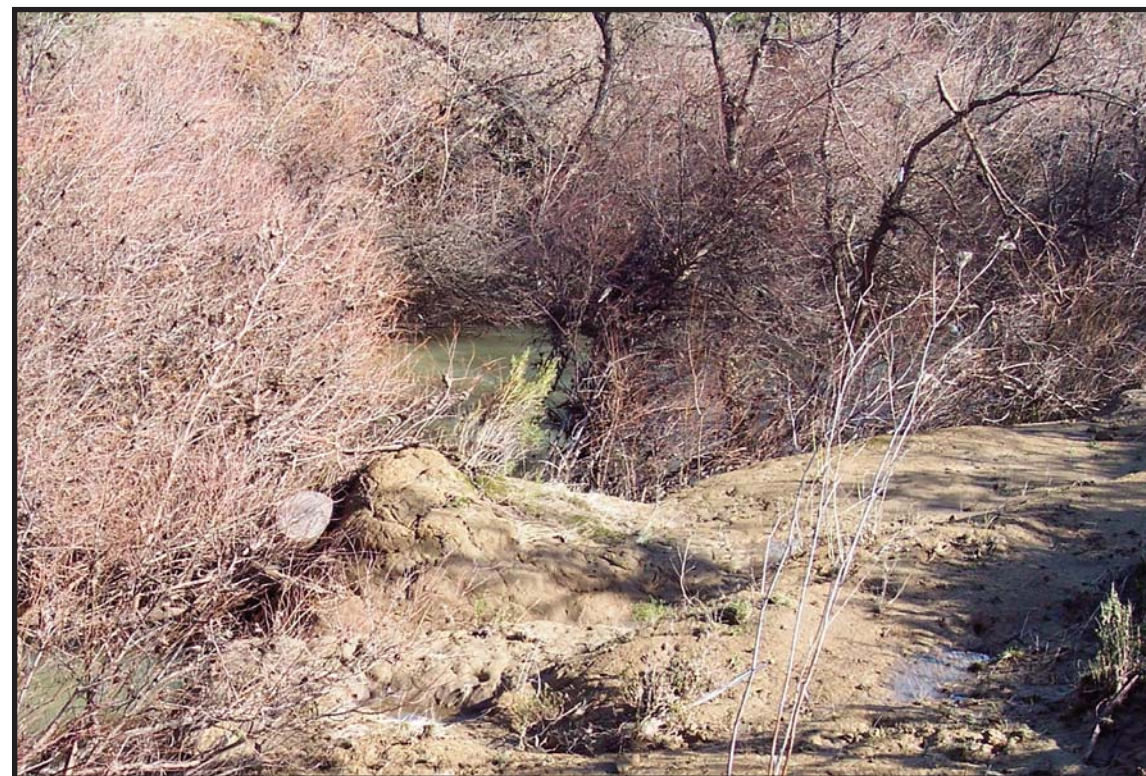
FAR LEFT: ENTRENCHMENT FROM THE NAPA RIVER HAS MOVED UP INTO DRY CREEK ERODING THE CHANNEL AND UNDERCUTTING TREES.
