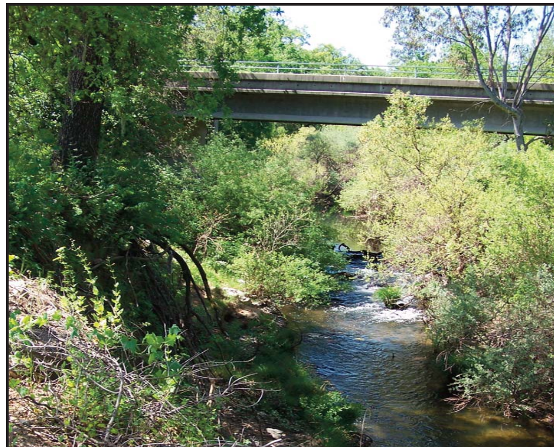
VIEW FROM AREA 18 LOOKING UPSTREAM AT YOUNTVILLE CROSS ROAD BRIDGE
