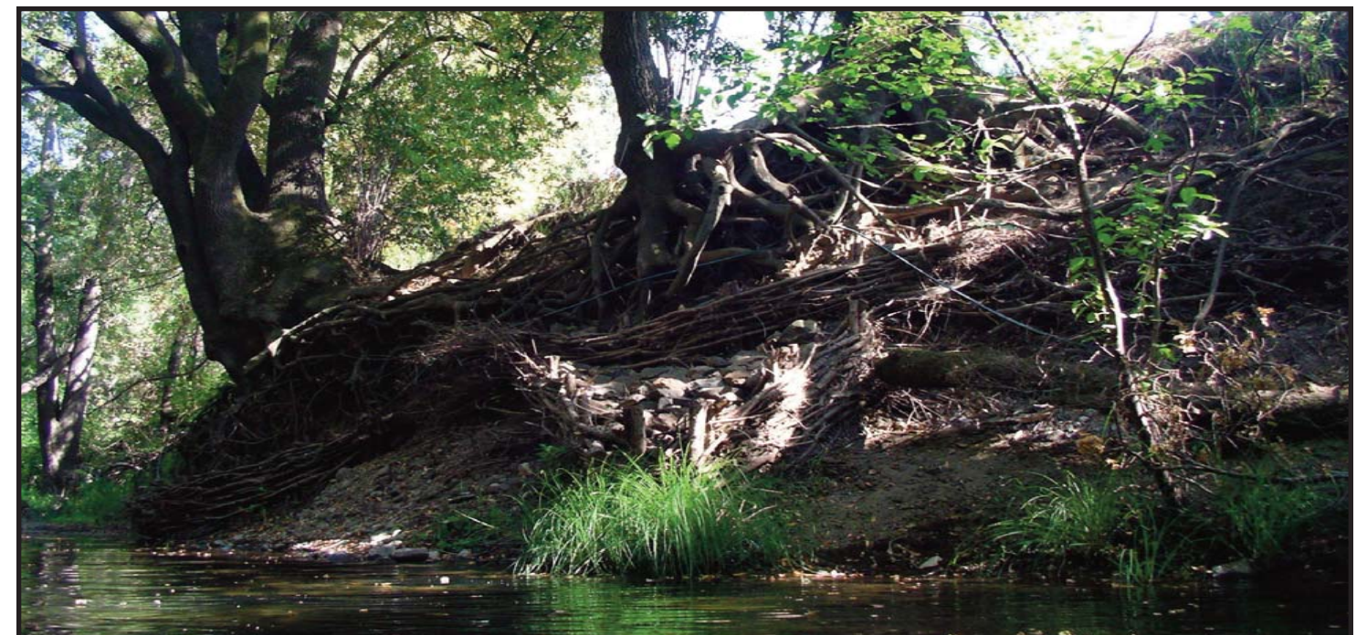
REACH 8 HAS NUMEROUS LARGE OLD GROWTH TREES. MANY OF THESE TREES ARE BEING UNDERCUT BY BANK EROSION. A WILLOW REVETMENT WAS CONSTRUCTED AROUND THE TREES IN THE PHOTO TO REDUCE EROSION BUT NEVER GREW.
