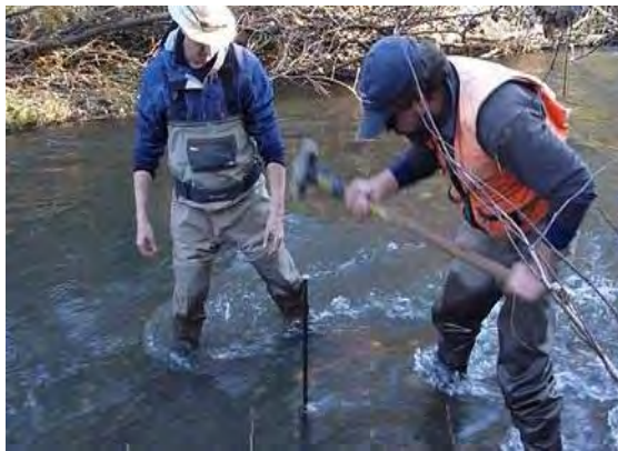
Installing a scour chain.
