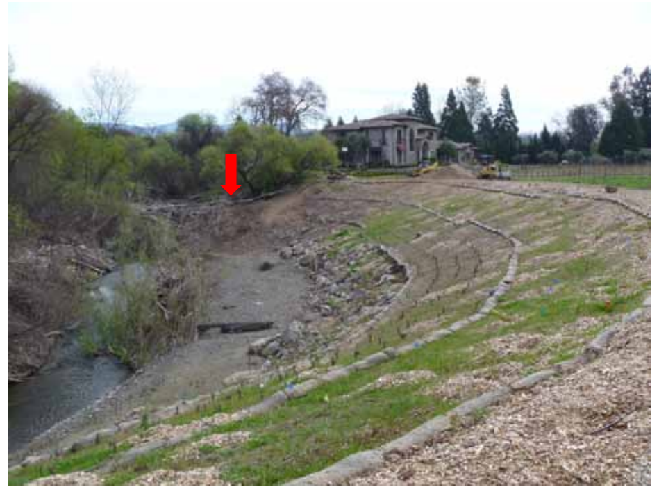
Figure 6: Large LWD jam January 2013 (after thinning)
