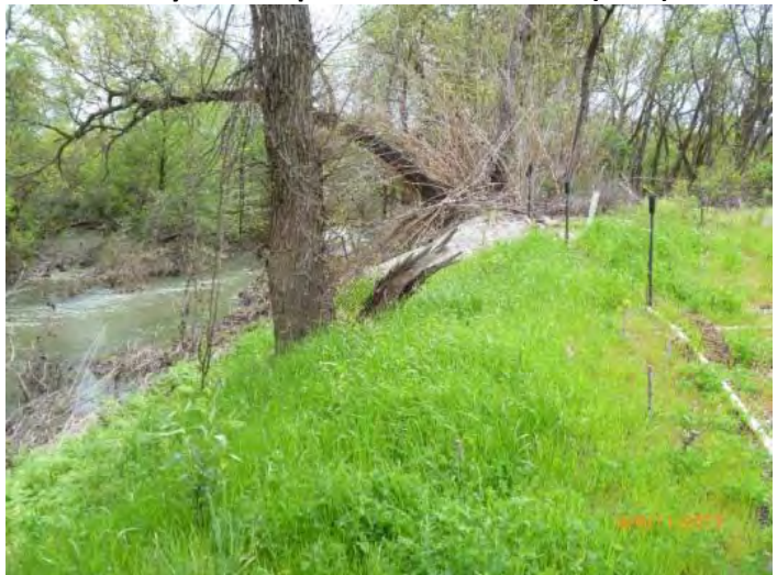
Picture 4: Caymus site post bank stabilization (2012)
