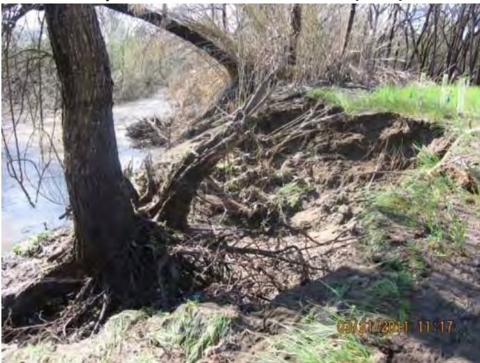
Picture 3: Caymus stream bank erosion site (2011)
