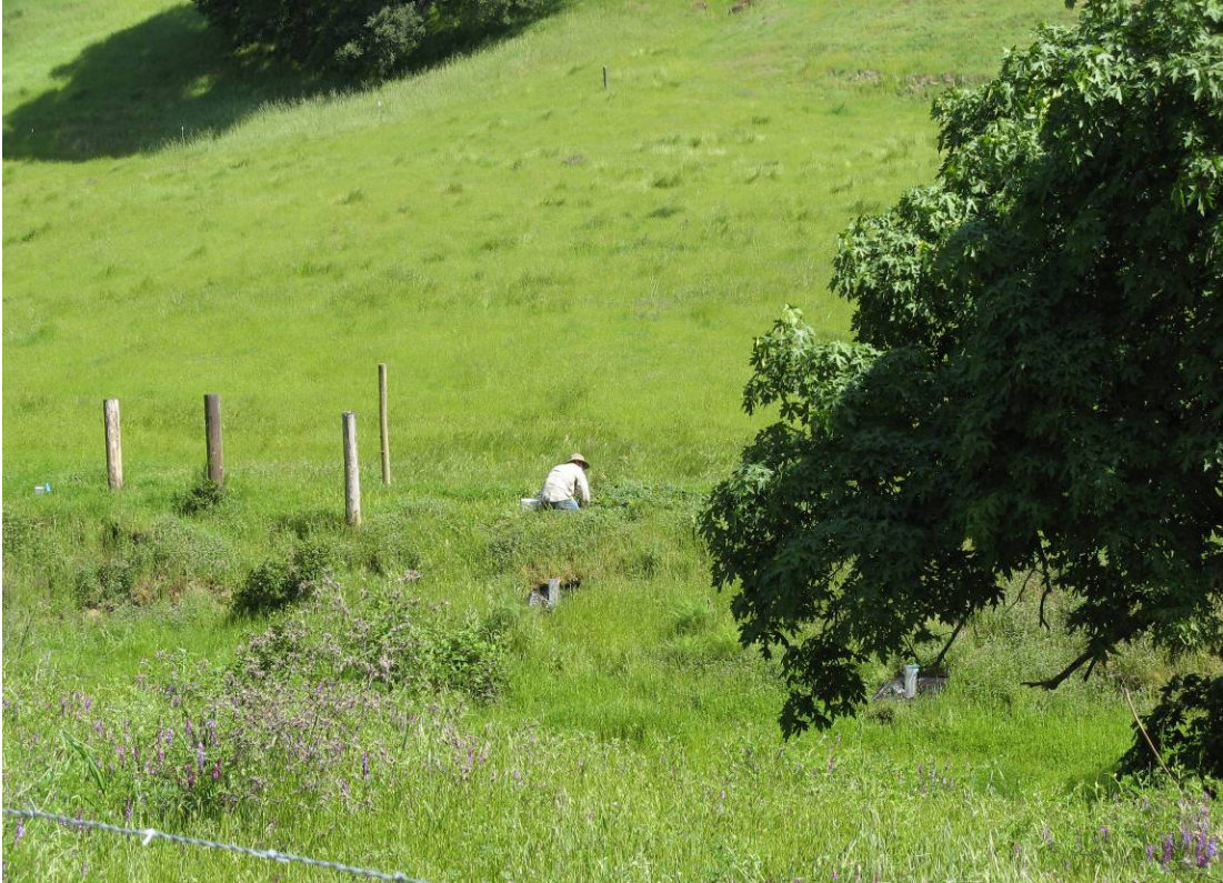
Figure 19: Wooden Valley Creek Riparian Habitat Enhancement Project – Plant Installation
