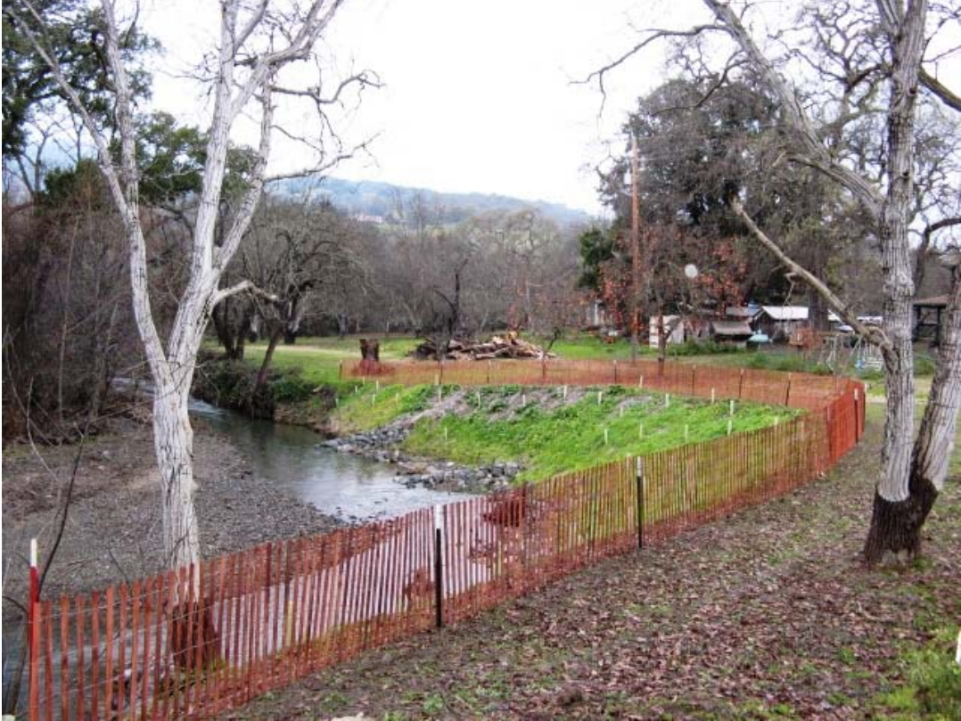
Figure 30: Suisun Creek Streambank Repair and Riparian Revegetation Project – After Project
