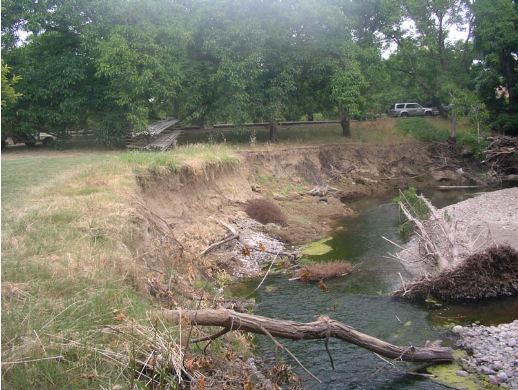
Figure 25: Suisun Creek Streambank Repair and Riparian Revegetation Project – Before Project
