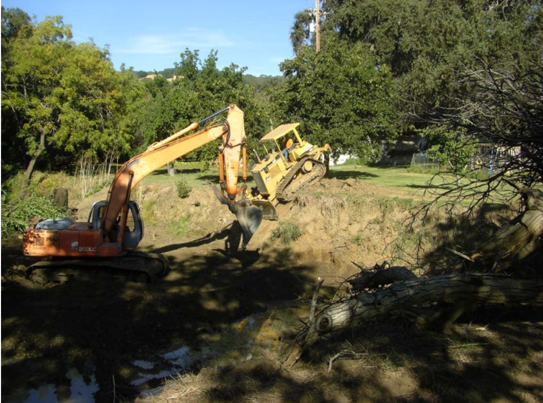
Figure 28: Suisun Creek Streambank Repair and Riparian Revegetation Project – Construction
