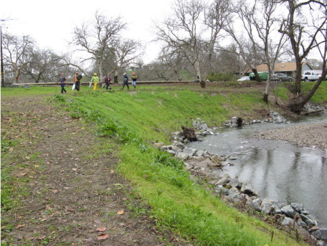
Figure 29: Suisun Creek Streambank Repair and Riparian Revegetation Project – Revegetation
