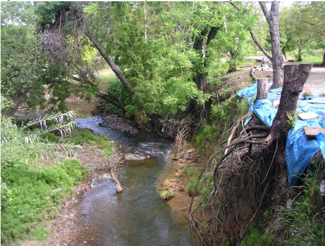
Figure 26: Suisun Creek Streambank Repair and Riparian Revegetation Project – Before Project
