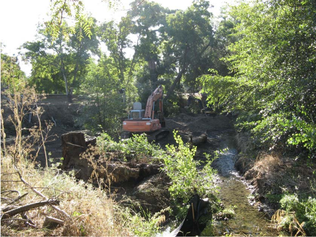
Figure 27: Suisun Creek Streambank Repair and Riparian Revegetation Project – Construction
