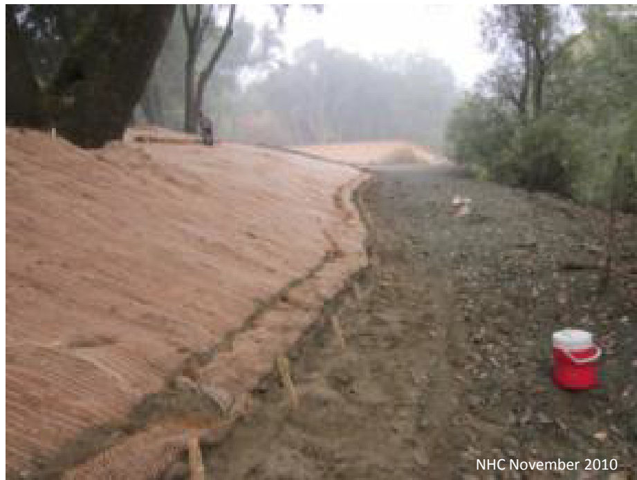
Looking Upstream from Station 21,750
