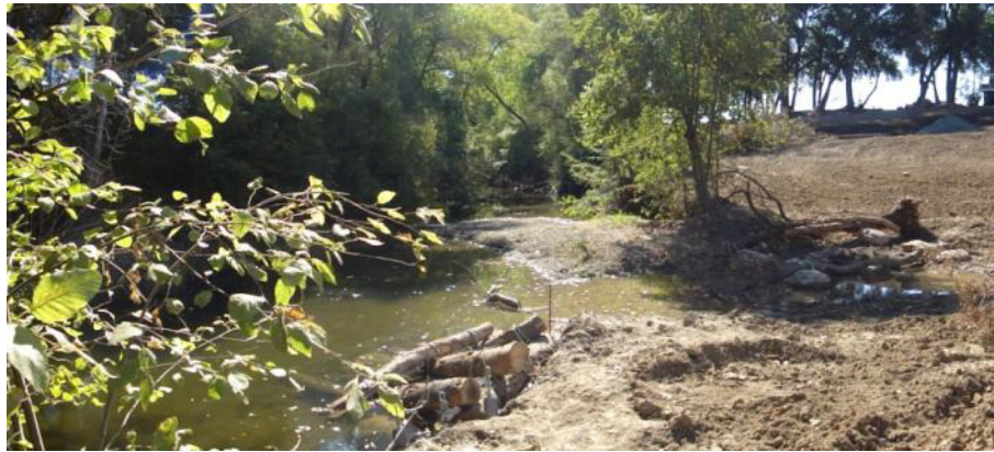
Looking Downstream From Station 22,200 to Station 21,100
