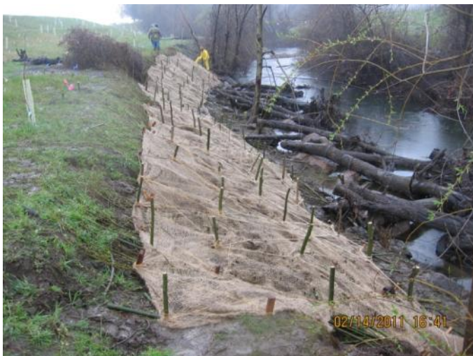
Picture 2: Installed willow brush mattress
