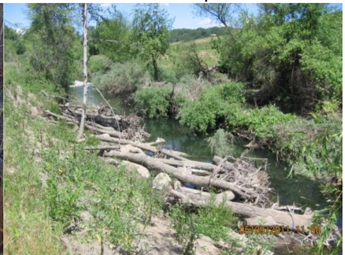
Picture 3: Brush mattress 3 month post installation
