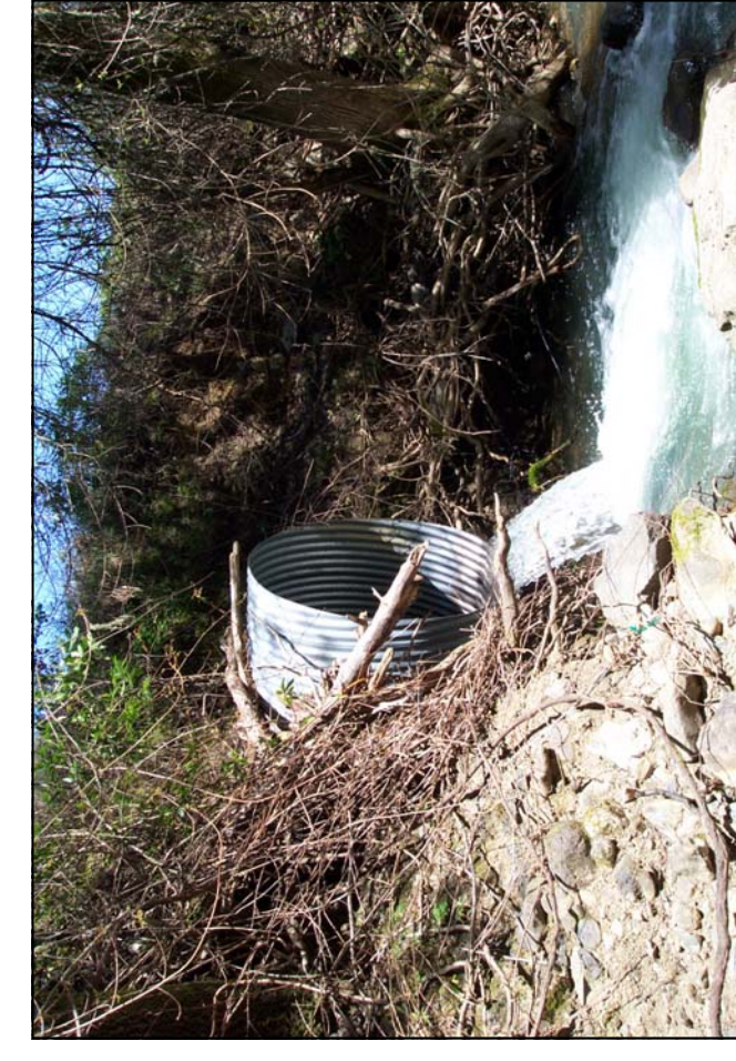
Dry Creek Road, Campbell Creek (trib to Dry)
