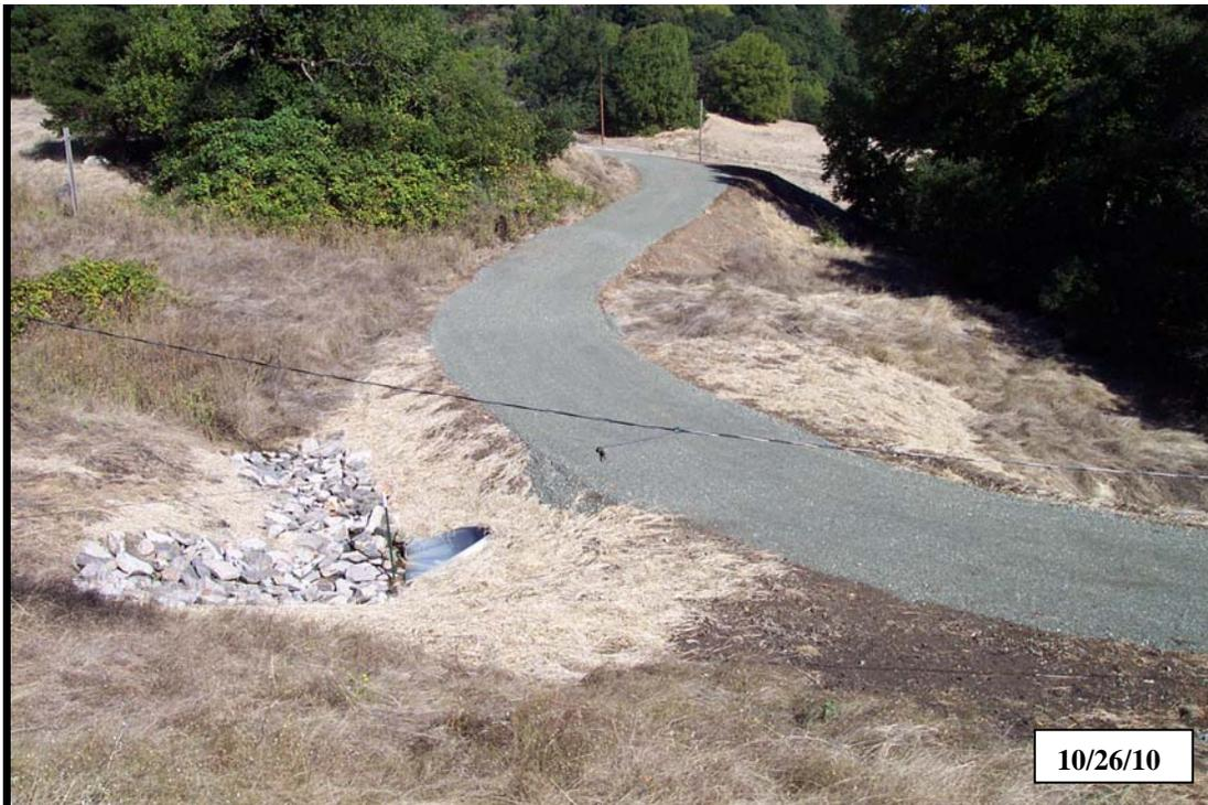
**Photo 7b.** Cain property, site #99, same view as above, after implementation. A new culvert with a flared inlet has been installed, as well as a trash rack. The inlet area has been armored with riprap, bare soil areas have been seeded and mulched, and the road has been re-rocked.
