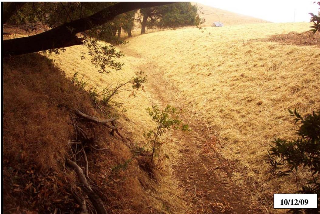
**Photo 3b.** Saintsbury property, site #200, same view as above, after implementation. The culvert has been removed, the channel excavated to natural grade, and channel banks sloped and mulched.
