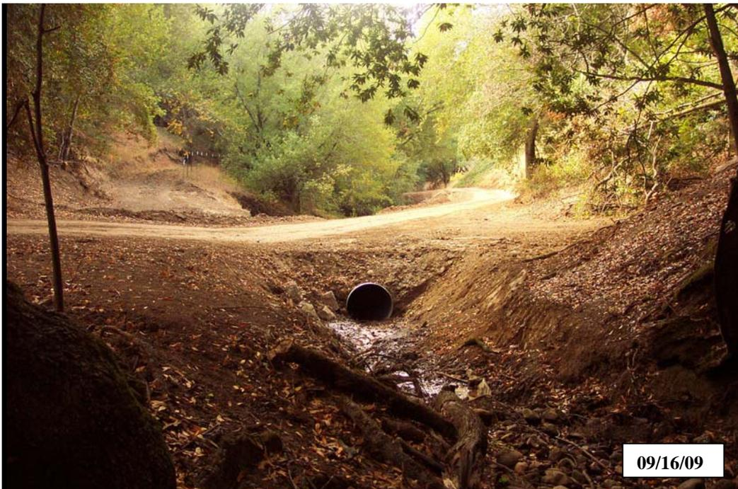
**Photo 1b.** Saintsbury property, site #180, same view as above, after implementation. A new 42 in. x 90 ft culvert has been installed at the base of fill
