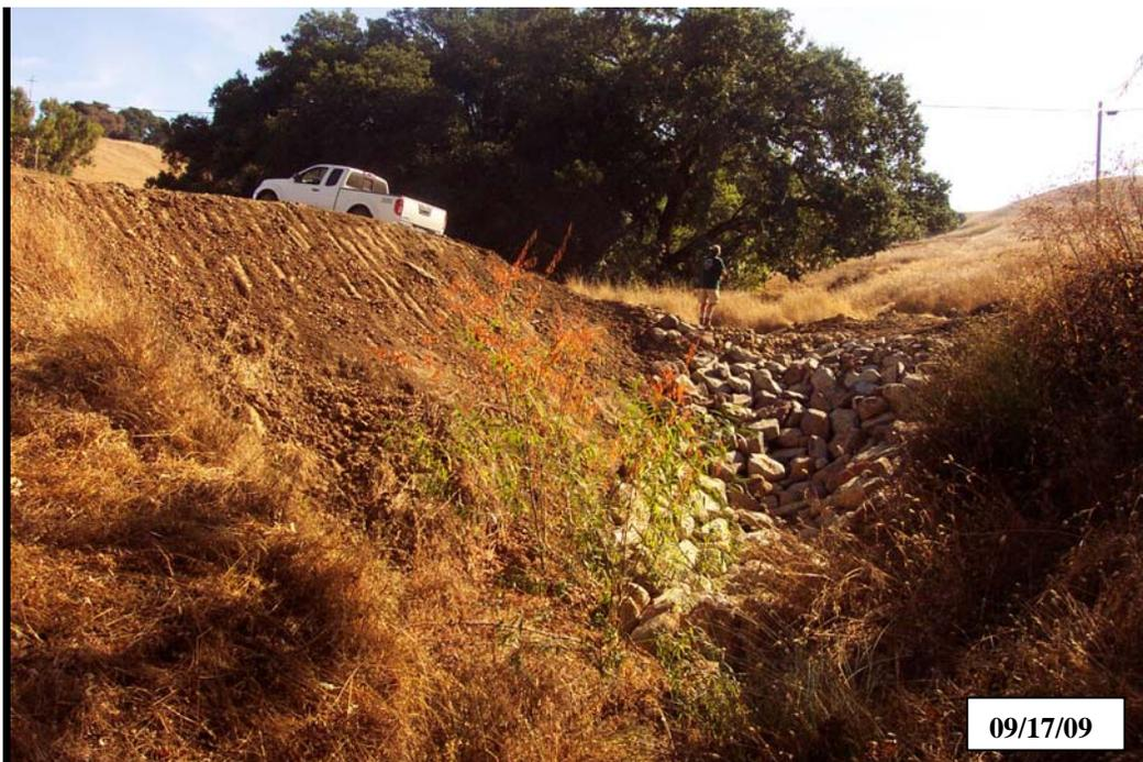
**Photo 2b.** Saintsbury property, site #197, same view as above, after implementation. An armored fill crossing has been constructed, and channel banks excavated back to stable angles and mulched.
