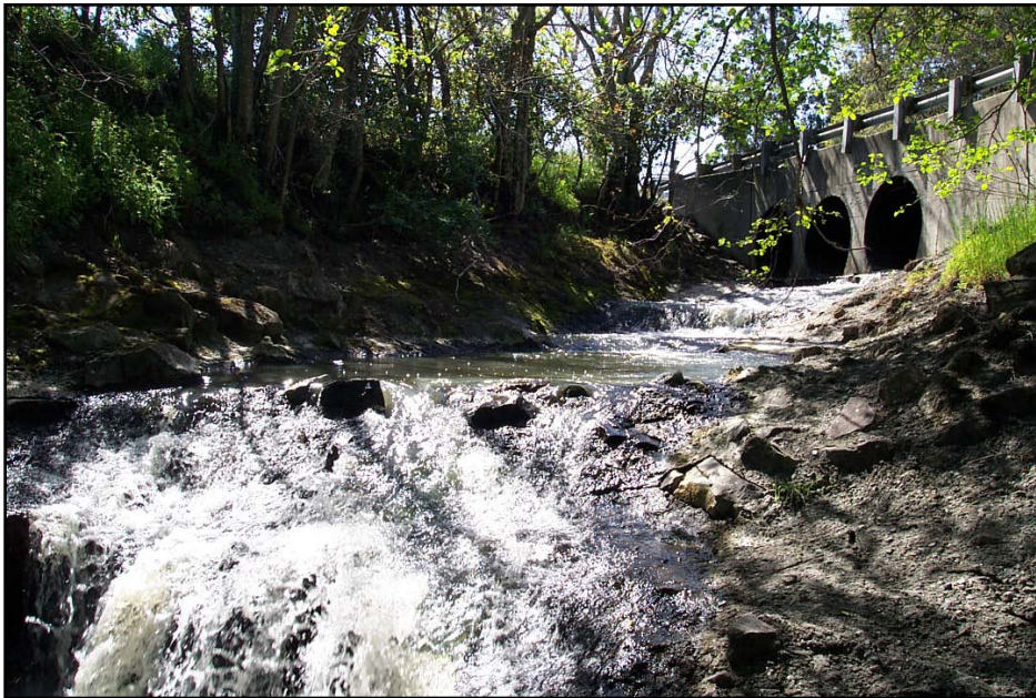
Highway 12/121 culvert crossing over Huichica Creek
