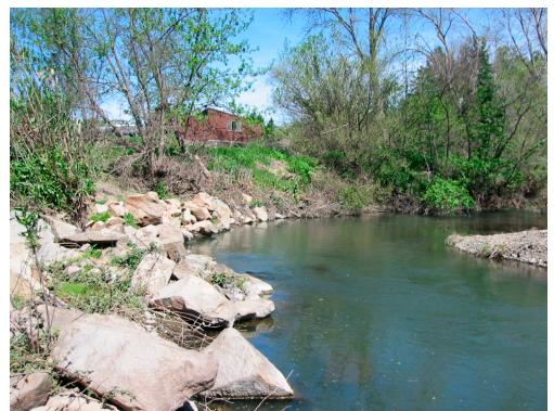
Photograph B-15. Undercut rip rap protection on the Wilsey property (west bank), stage 5 outside bend
