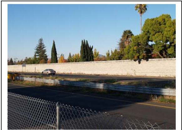
A sound barrier must block the line of sight between the source and receiver to provide attenuation of the direct sound.
