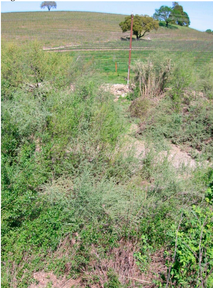
Photograph B-46. Bank erosion on the Quintessa property, from mid way up Frogs Leap
