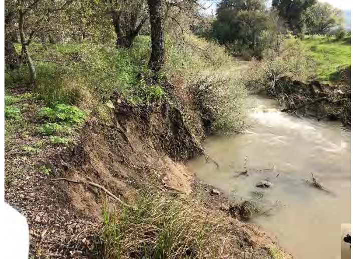
Picture 2: Bank Erosion Site reach 8
