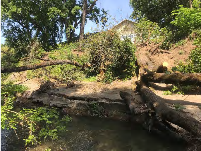
Picture 1: Bank Erosion Site Reach 8
