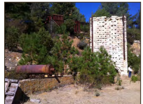
Decaying ore processing structures
