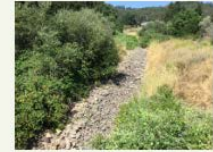
The creek bed is completely dry, there is no water.
