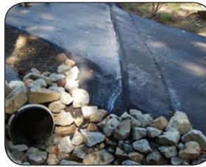
**B** A small speed bump known as a waterbar can be added to existing driveways to SLOW and SPREAD runoff to vegetated or rocked infiltration areas (page 43).
