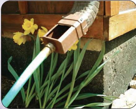
**SPLASH GUARDS** are simple devices that reduce the initial force of the water at the outlets and allow it to SPREAD out into an area of vegetation or an appropriate infiltration area and SINK back in to the soil.
