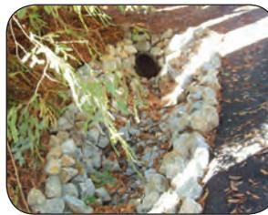
**D** A rocky or vegetated swale lining the edge of a road or driveway reduces erosion potential by SLOWING runoff and then SINKING it back into the soil or directing it to a safer outlet (pages 34-35).
