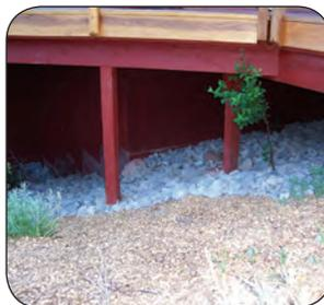
**B** Adding drain rock SLOWS runoff and safeguards the drip-line area under elevated surfaces. Mulch around the perimeter adds extra protection to the surrounding bare soil (pages 27-28).
