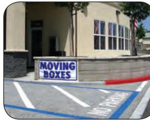
**C** Pervious concrete (pictured) or other materials such as paver stones or turf block, allow water to SINK into the soil decreasing runoff (pages 38-39).
