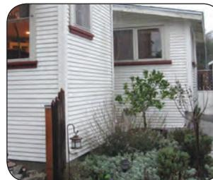
**B** Vegetated or rock drip-line protection SLOWS runoff thus reducing erosion and promoting infiltration. It is also designed so that the ground slopes away from the home's foundation (see page 27)
