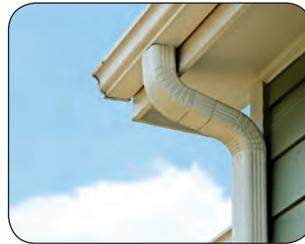
**A** Adding gutters and downspouts works to direct water to a safe location away from bare soil and buildings (see page 25).
