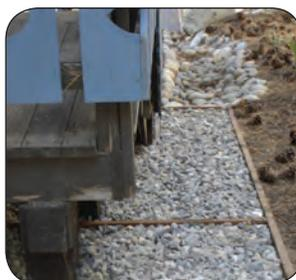
**A** Adding drain rock or vegetation to the perimeter SLOWS and SPREADS water limiting the transport of sediment (pages 27-28)
