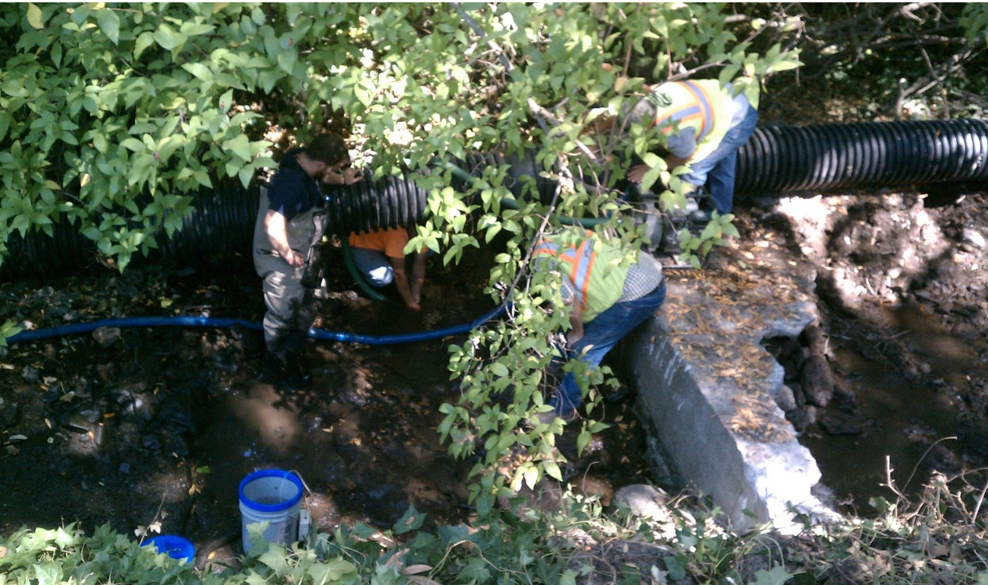
In the process of dewatering the creek and capturing and relocating fish and crayfish.
