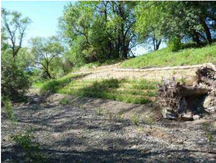
Picture 3: Reach 8 erosion repair site (March 2013)
