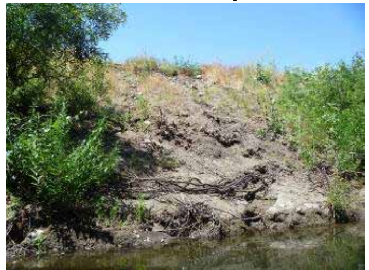
Picture 4: Arundo treatment site showing bank erosion
