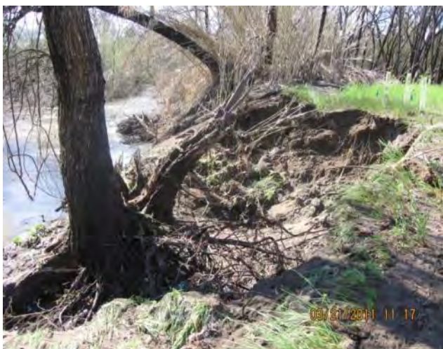
Figure 5: Erosion at constructed bench (before)
