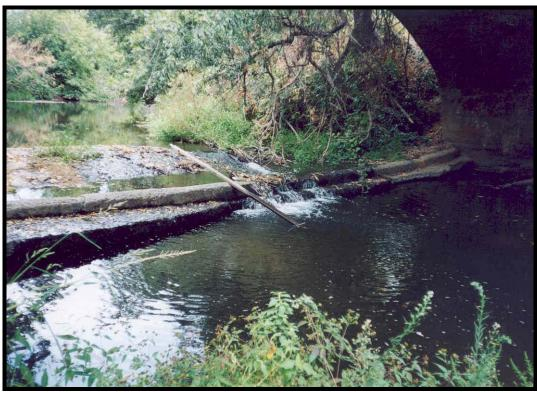
Station Suisun Creek 4 (SC4) — Note cement drop structure under bridge
