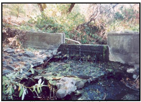
Old concrete structure on Wooden Valley Creek — may be blocking fish passage downstream of WV3
