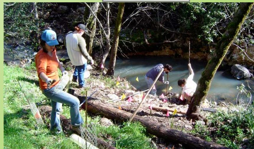
**Restoration focuses on increasing protective vegetation** on highly erodible stream banks to reduce sediment supply and increase channel stability.
