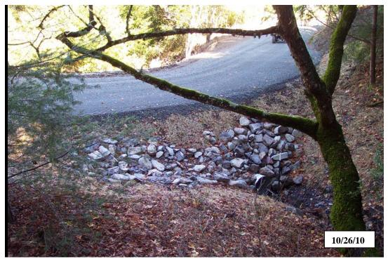
**Photo 5b.** Cain property, site #54.1, same view as above, after implementation. A new 24 in. x 70 ft culvert has been installed at the base of fill and a trash rack placed upstream from the inlet. Also the road surface has been re-rocked.
