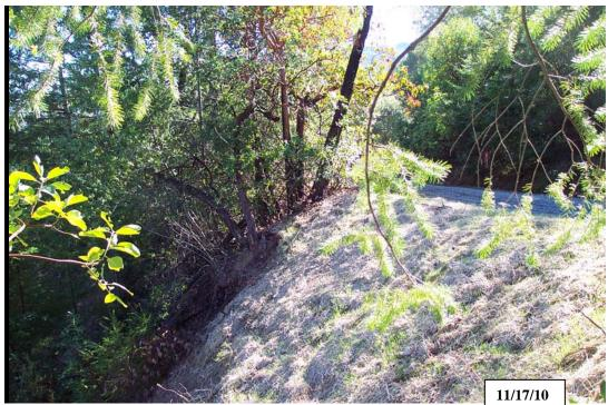
**Photo 8b** Marston property, site #2001, same view as above, after implementation. Oversteepened and perched material has been removed. Bare soils have been seeded and mulched with straw.
