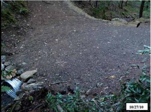
**Photo 9b** Hoffman property, site #133, same view as above, after implementation. A new, properly sized oval culvert has been installed at the base of fill in alignment with the natural channel. A trash rack was installed above the inlet.
