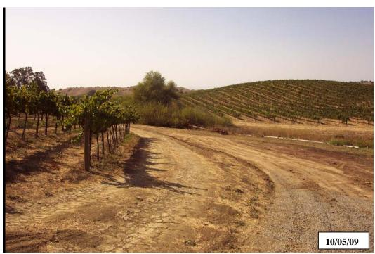
**Photo 4b.** Artesa property, site #217, same view as above, after implementation. A rolling dip has been constructed to disperse road drainage and reduce the amount of concentrated runoff reaching the stream.
