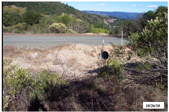
**Photo 6b.** Cain property, site #55.1, same view as above, after implementation. A new culvert and trash rack have been installed, and the road surface has been re-rocked.
