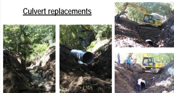
Culverts installed at base of fill and adequately sized
