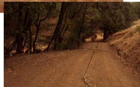
3% to 4% road outsloping with no ditch or berm drains vineyard and road runoff into vegetation
