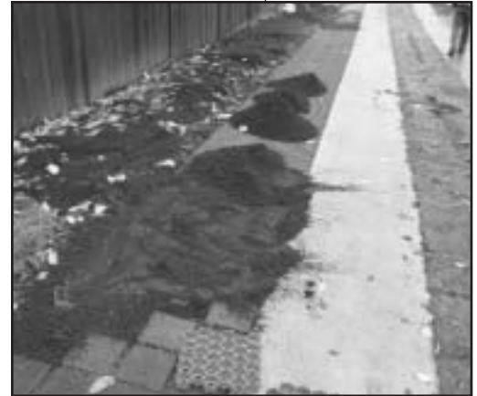
Preparing structural grass.
