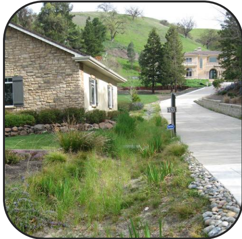
Large Residential Rain Garden
