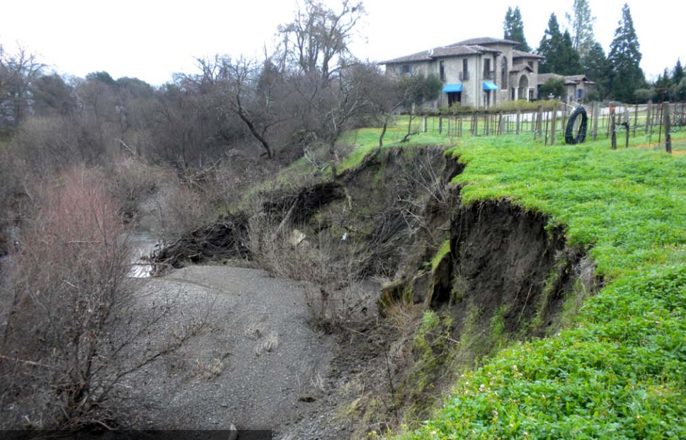
Sequoia Grove pre construction
