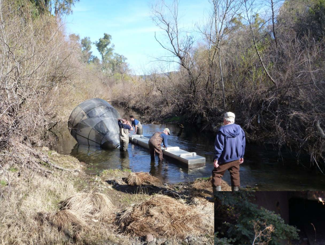
Volunteers constructing and installing Napa River rotary screw trap
