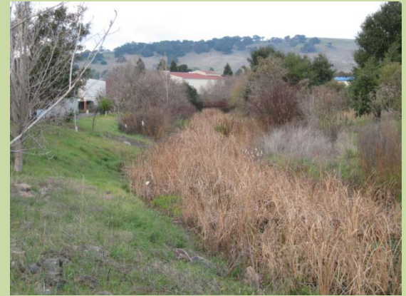
Sediment and cattails at Sheehy Cr.
