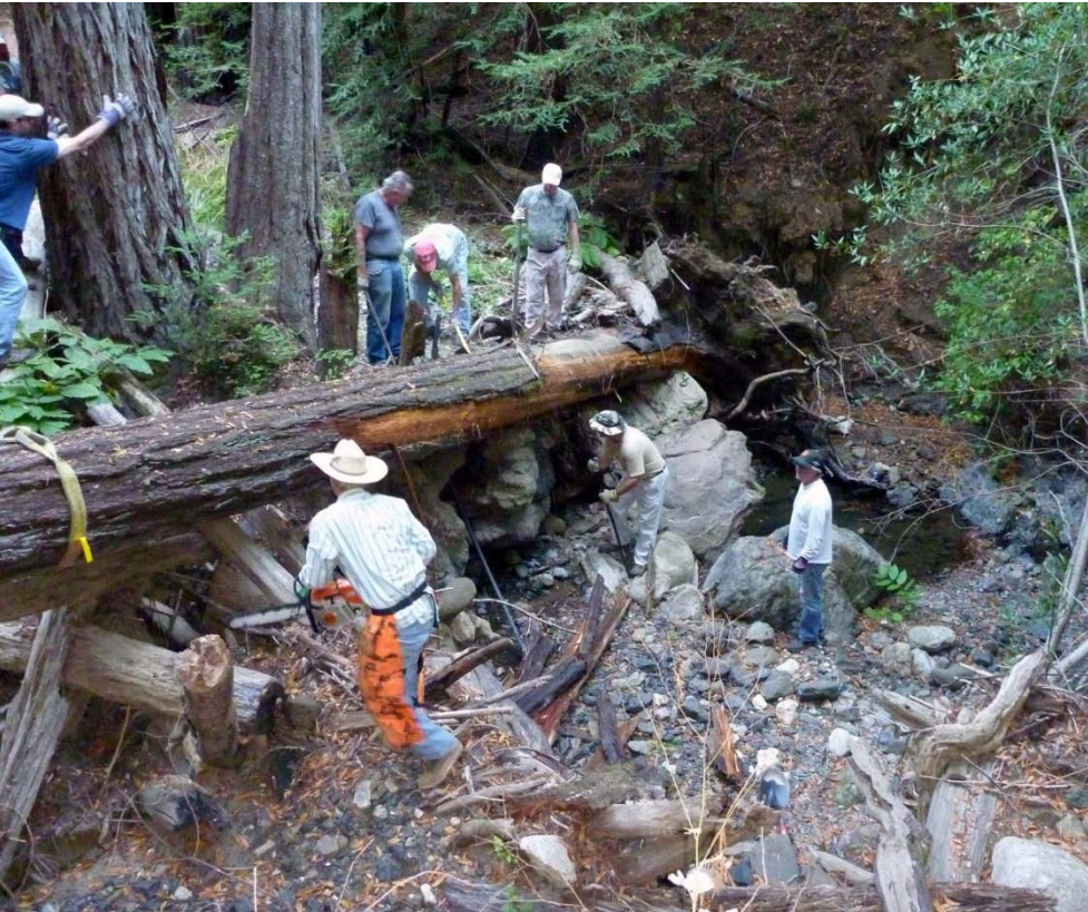
Volunteers removing fish passage barrier from Wing Canyon Creek
