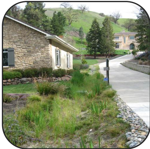
Large Residential Rain Garden
